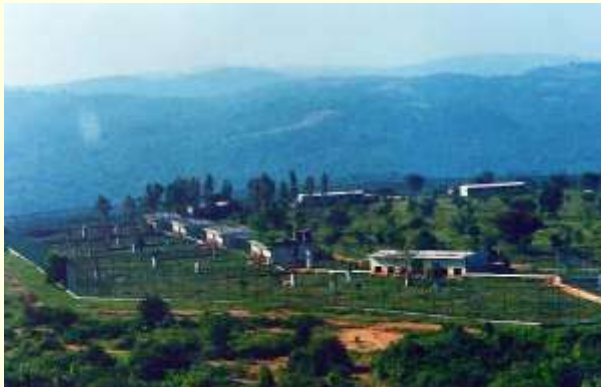
Rescue center - overview
